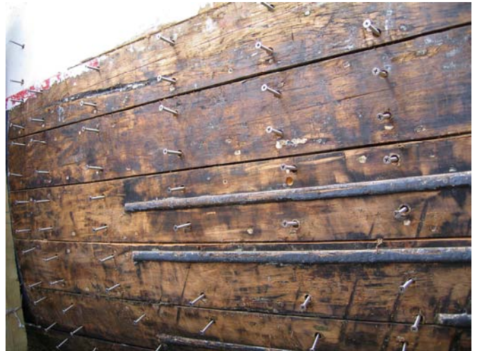
Screws in place ready for driving
