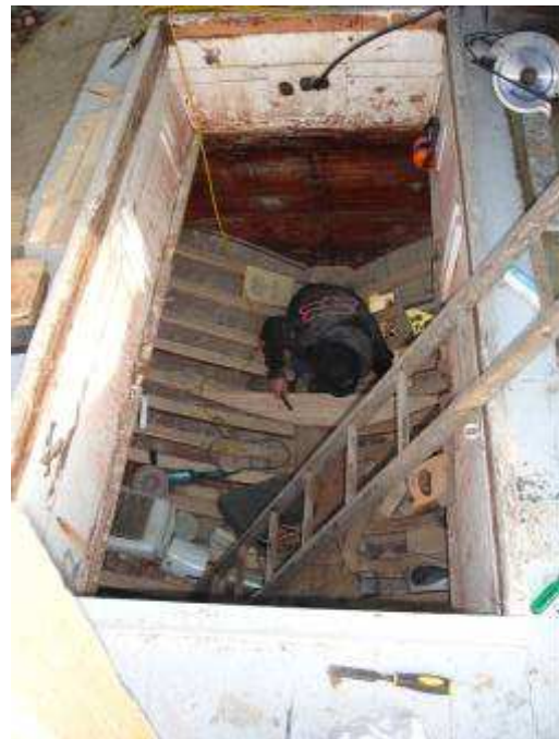
A new keel top, more ribs and new floors were installed in the well.
