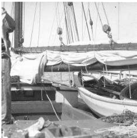
The gaff, mainsail and boom of the original rig
